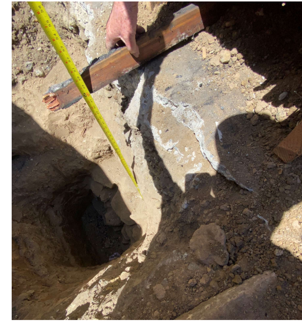
Top of Grade to Top of Culvert - 48"
