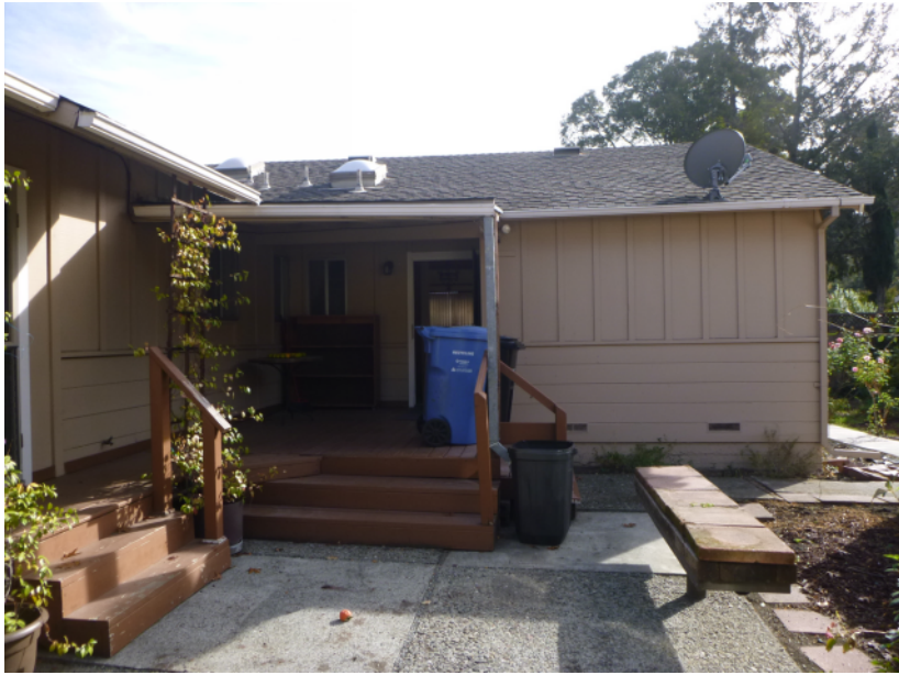
REAR DETAIL - PORCH
